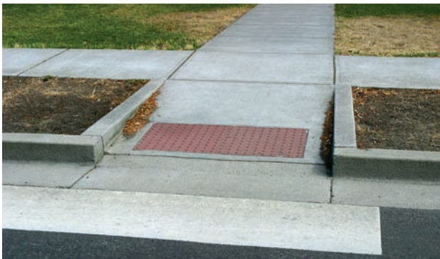
Perpendicular Curb Ramp
