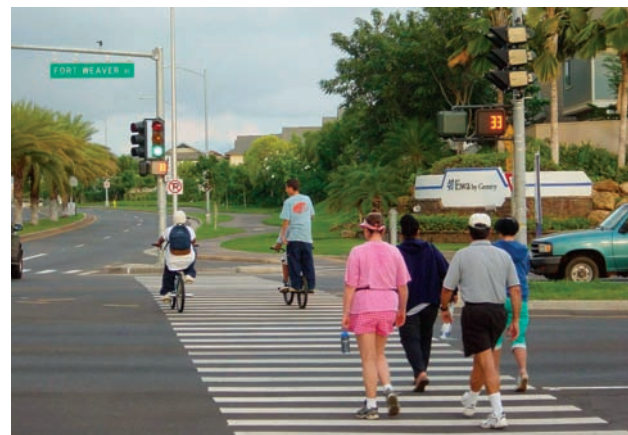
Pedestrian signal head in line with crosswalk
