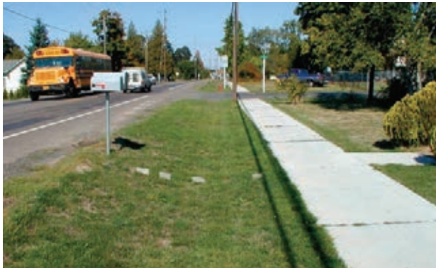
Sidewalk behind swale
