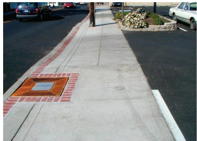
Dustpan style driveway approach improves pedestrian safety
