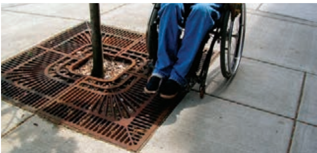
Wheelchair traversable tree grates may extend into pedestrian zone
