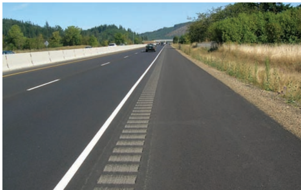
Well placed rumble strip leaves room for bicyclists
