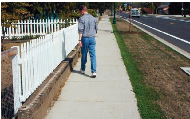
Sidewalks serve pedestrians in urban and suburb contexts
