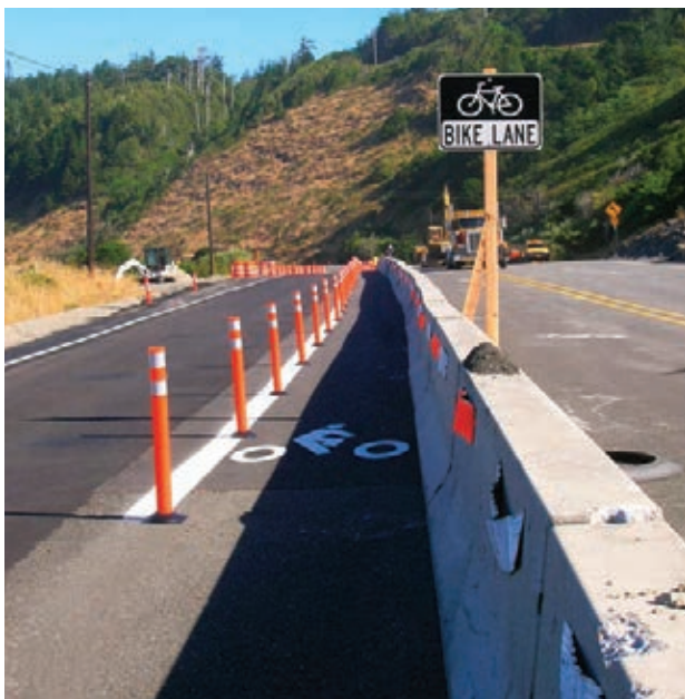
Bike lane in temporary work zone
