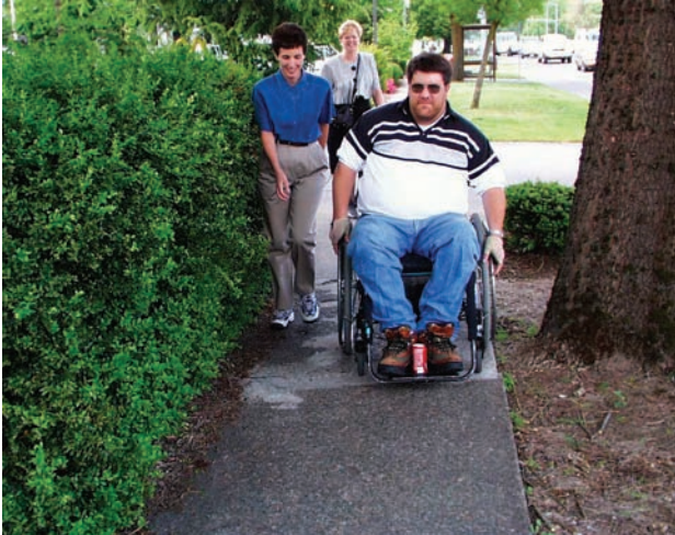
5 foot sidewalk is uncomfortably narrow
