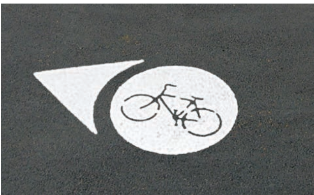
1st Generation bicycle boulevard pavement marking
