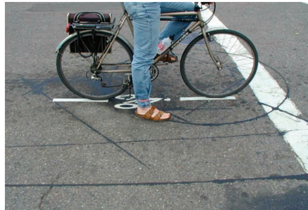
Stencil indicates where to position bicycle over loop detector to trip signal
