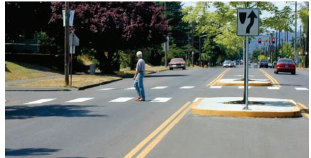
Median island provides mid-street refuge for pedestrians
