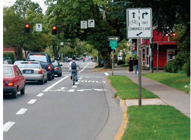
Combined right turn lane and thru bike lane
