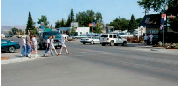
Motorist yields to pedestrians at curb extension
