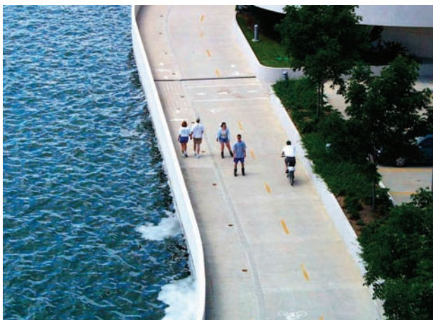
Path striped to separate users
