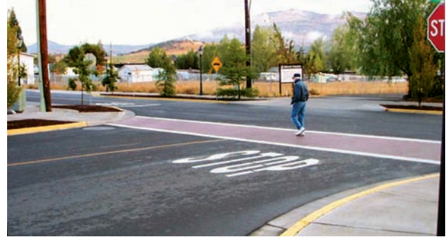
Textured crosswalk with supplemental white markings
