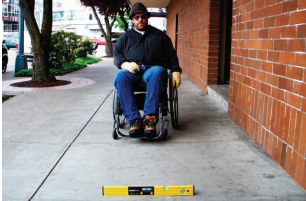
Steep cross slope (4%) is difficult to traverse in a wheelchair
