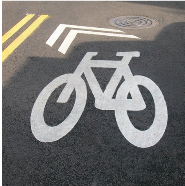
2nd Generation bicycle boulevard pavement marking (indicates turn)
