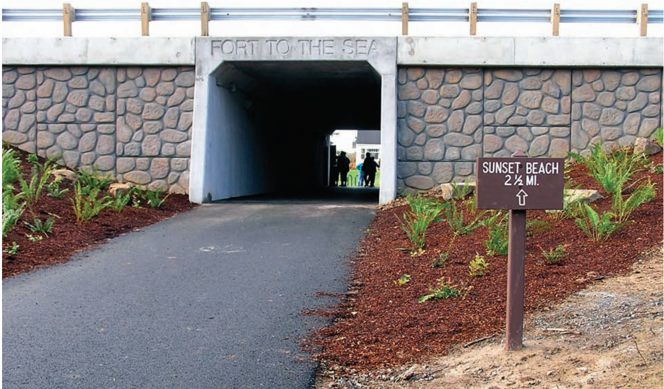
Undercrossing with good sight lines
