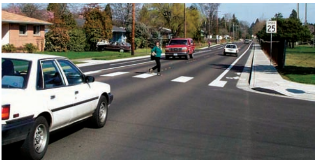
Painted crosswalk on two lane roadway is appropriate
