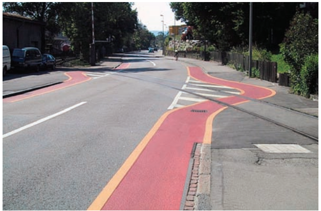
Rail crossing S curve
