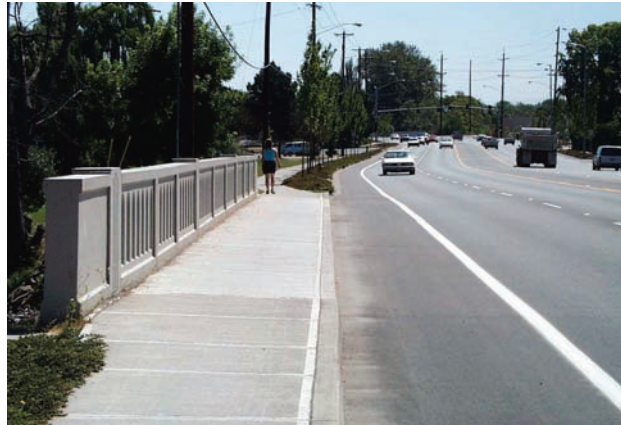
Furniture zone eliminated at pinch point
