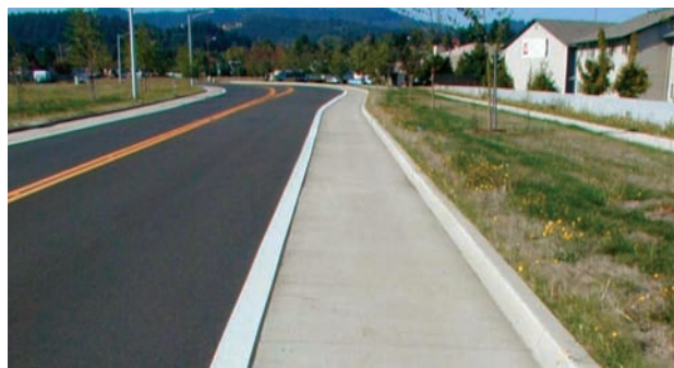
Concrete bike lane provides contrast with asphalt roadway
