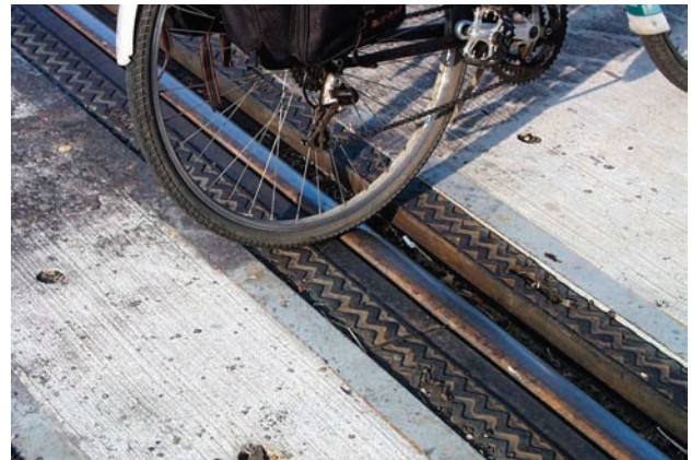
Concrete RR crossing with rubber flanges
