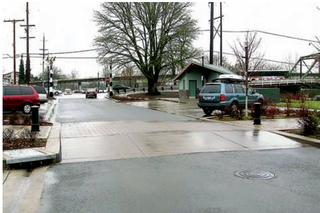
Raised intersection keeps crossing level with sidewalk
