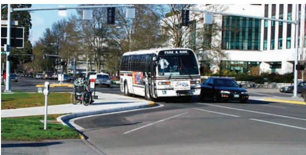
Curb extension bus stop reduces bus dwell time
