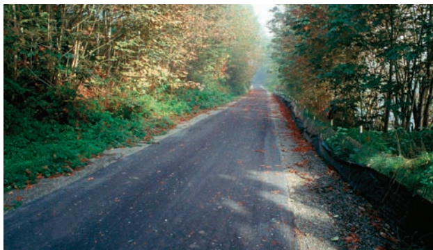
Gravel shoulders prevent raveling of path edges
