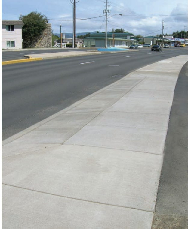
Wide sidewalk accommodates driveway and keeps pedestrian access route level
