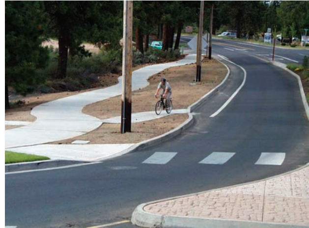
Bicyclist using exit ramp to access sidewalk
