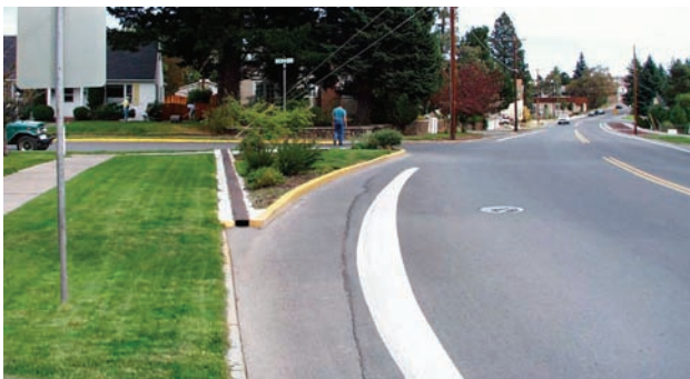
Formerly skewed intersection realigned to right-angle
