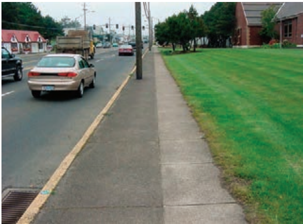
Sidewalk widened to 6 feet
