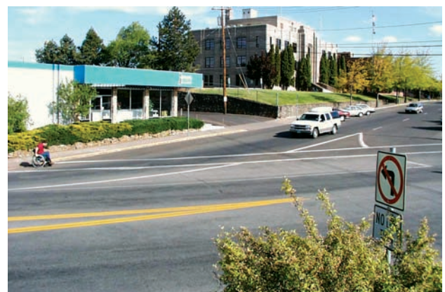
Skewed intersection results in long crosswalk and increased pedestrian exposure
