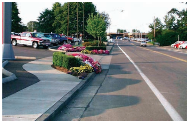
Sidewalk is kept level at driveway
