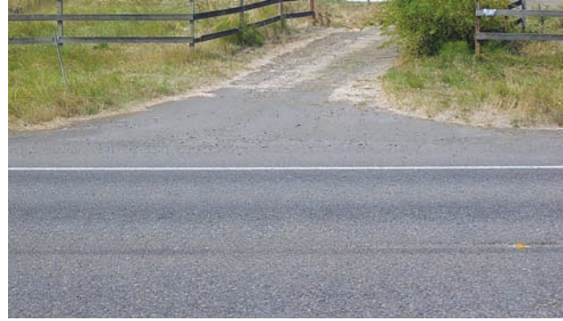
Paved driveway apron keeps gravel off shoulder
