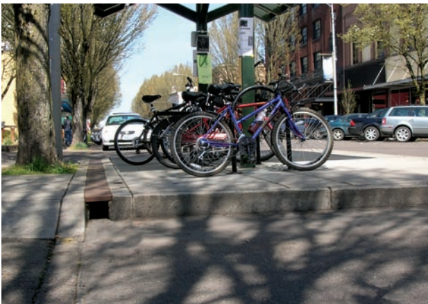
Slotted drain at retrofit curb extension
