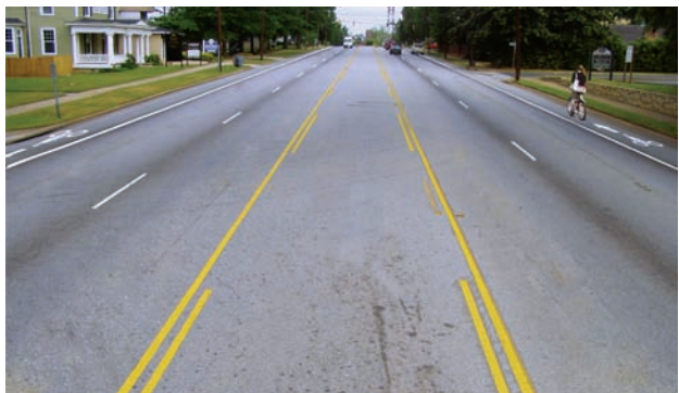
5 lane roadway with bike lanes, narrowed motor vehicle lanes
