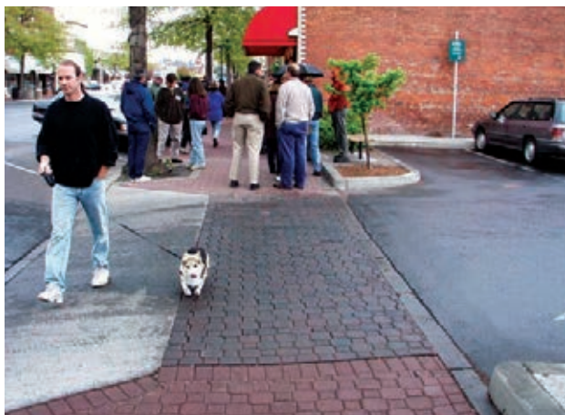
Sidewalk thru alley entrance is kept level
