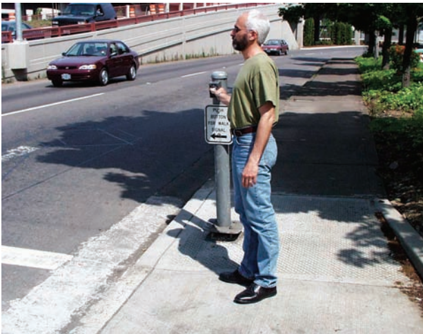
Pushbutton placed and aligned for the visually impaired
