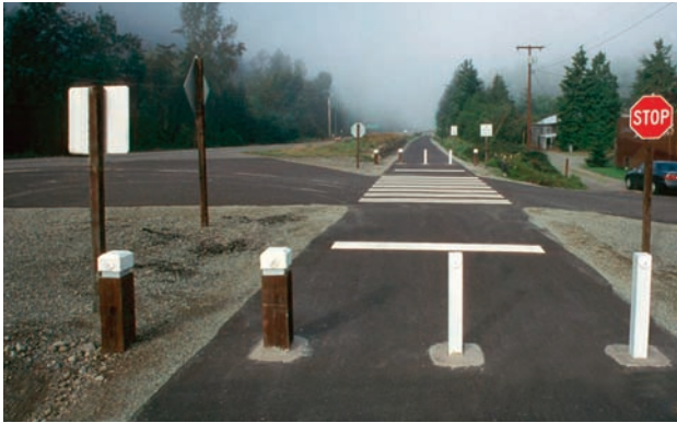
Path crossing a minor street should have been given priority right of way
