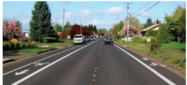
Parking removed from one side to add bike lane
