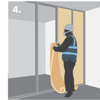
4. Inserting Knauf insulation quilt between the Knauf 'C' or 'U' Studs.
