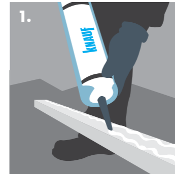
1. Applying two continuous beads of Knauf Sealant to perimeter framing.
