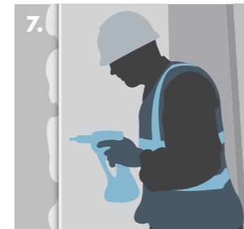
7. Fixing Knauf Plasterboard onto the Knauf Metal Furring Channel.
