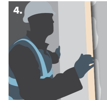
4. Offering up Knauf Insulating Laminate for a better thermal performance.
