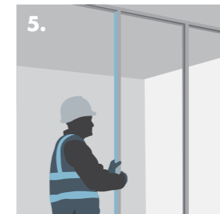
5. Inserting timber ground into jamb stud door opening.
