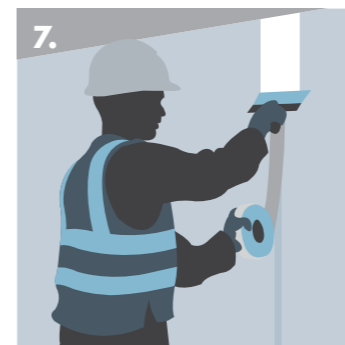
7. Taping and jointing for a seamless finish.
