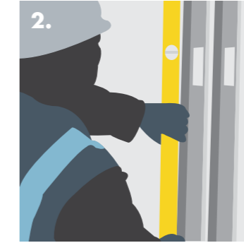
2. After fixing the head track, the floor track should be positioned by using a vertical stud and a spirit level.
