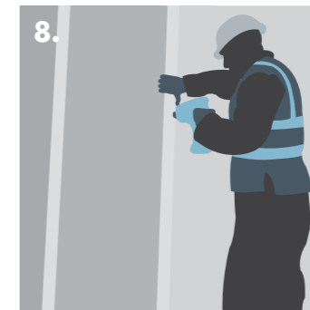
8. Fixing Knauf Plasterboard to the completed framework.
