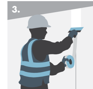
3. Embedding Knauf Aquapanel Exterior Joint Tape.
