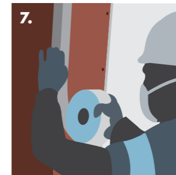
7. Taping and jointing encasement corners
