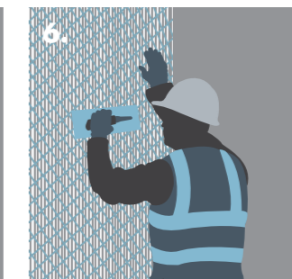
6. Applying reinforcing mesh.
