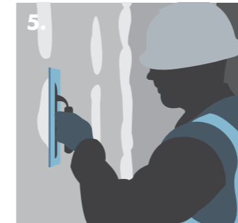
5. Applying Knauf Plasterboard Adhesive around the perimeter and at the required centres.
