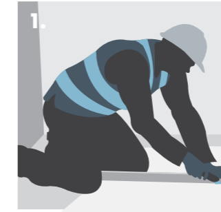
1. Scoring Knauf Aquapanel Exterior with a knife.
